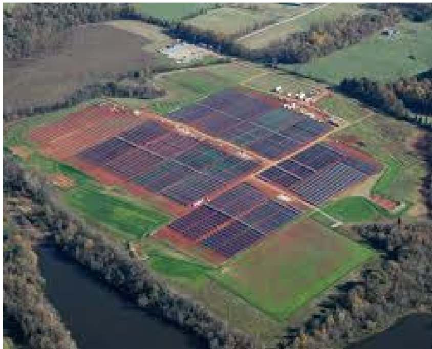
Figure 2. Thirty-acre solar facility in western North Carolina.
